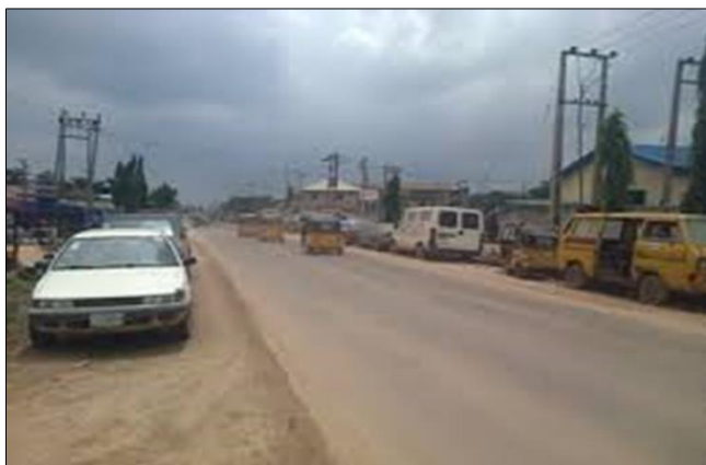
Fig 5: New layouts are opening up without requisite infrastructural layout. A new estate without drains.
