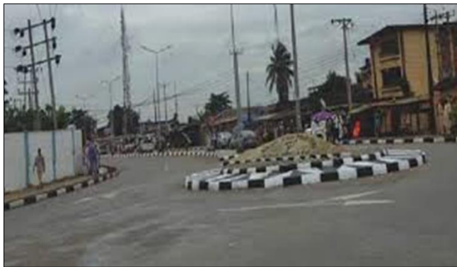
Fig 6: Road upgrade to create better access
